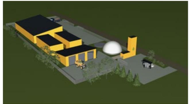
BioGTS® Biogas plant, feedstock 10 000 t/y, 27 t/d of agricultural biomass
